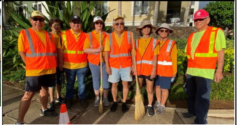
HK Lions repairing sidewalks along Wailua Street.
