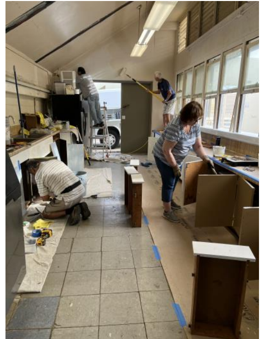
Kaiser High School Concession Stand (Work-In-Progress)
